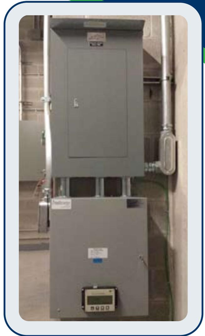
It combines a three phase distribution panelboard with 250 Ampere bus bars and 12 two pole breakers for 208 Volts rated 40 amps, a Measurement Canada approved i-meter 45, an individual contactor for each charger circuit and a controller that is programmable to set a timer for each charger.
