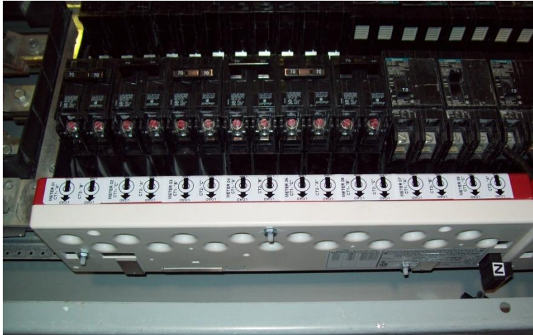
Typical i-meter™ 636 INC Installation
