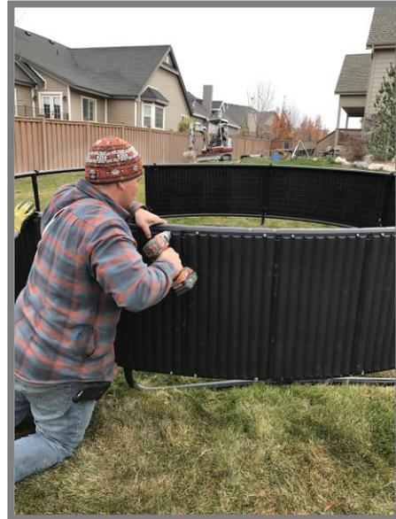
6. At this point- slide together the remaining 10 panels \*without securing them to the frame, and insert/secure the final panel to the first panel by sliding the joints together.
