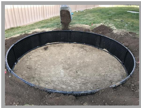
12. Be sure to backfill evenly around the trampoline frame- by filling in 1ft. lifts all the way around the trampoline, and then adding the next 1ft. lift all the way around the trampoline until complete.
