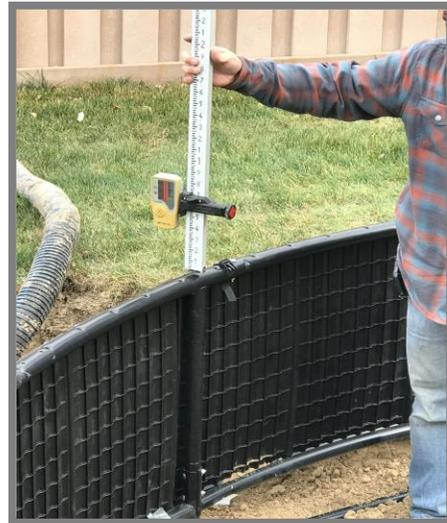
10. Begin backfilling the inside of the Trampoline Hole by placing excess soil at the base of the trampoline retaining wall.
