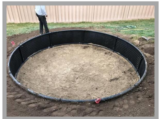
13. With the interior and exterior of the hole properly backfilled and compacted- you are now ready to install the jumping mat, springs, and Vented safety pad.
