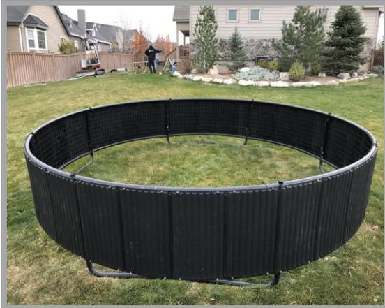
8. With your Trampoline Frame and Retaining wall complete- you are now ready to set the system in the previously dug hole. With the help of 1 or 2 people- lift the system into the center of the hole.
