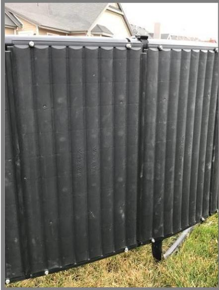
4. Continue placing screws in the remaining 3 Screw bases on the 1st panel in the following order: 1<sup>st</sup> upper right, 2<sup>nd</sup> lower right, 3<sup>rd</sup> lower left, 4<sup>th</sup> upper left.
