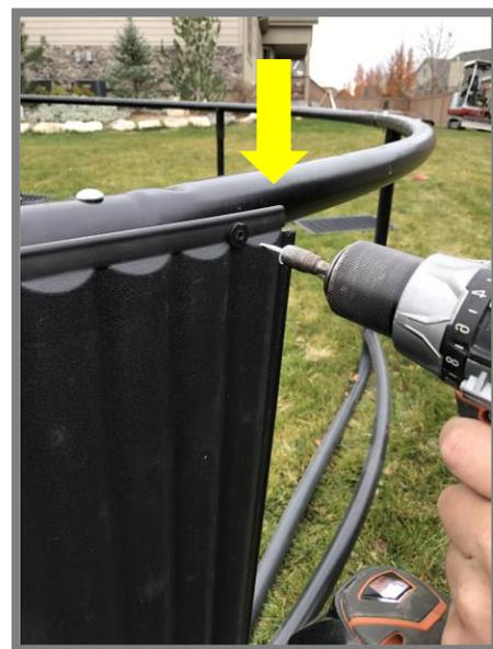
Secure the first panel by placing a Screw in the upper right screw location on the panel. (as shown above in figure 1)
