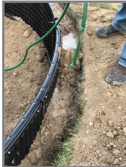
**\*\*NOTE:** Do not use a tractor to drive around the trampoline to compact the soil- and be cautious using a jumping jack- as excessive compaction force can potentially damage the Trampoline Frame, or push it out of round.
