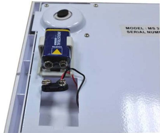
Intalling 9V battery
