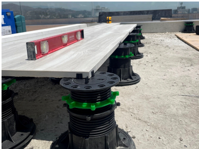
Pedestal Installation Method
