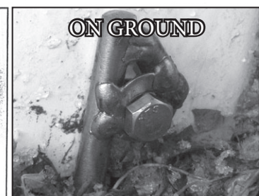
4 Stainless Steel Anchors 4 Lag Bolts
