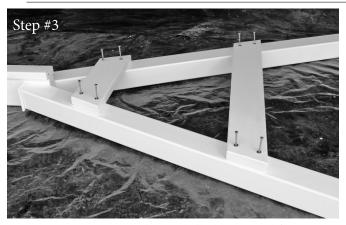
A. Line up Braces with the predrilled holes and fasten using  $^{1}\!4$ " x 4" Lag Bolts with a Washer. B. In the event that your A-Frame does not include a Vinyl A-Frame Roof, insert the two Vinyl Hole Plugs into the extra predrilled hole.
