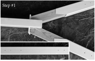
Fasten legs using 3/8" x 7½" Machine Bolts (on both sides of swing). <u>Note:</u> Two of the legs will have five (5) predrilled holes (see inset). Make sure one of these legs is located on each end of structure.
