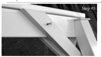
Fasten the Top Braces to the Top Beam using  $\frac{5}{16}$ " x  $\frac{51}{2}$ " Machine Bolts and  $\frac{5}{16}$ " Washers & Flange Nuts.
