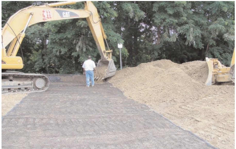
Mirafi® BXG biaxial geogrids are installed for base reinforcement.
