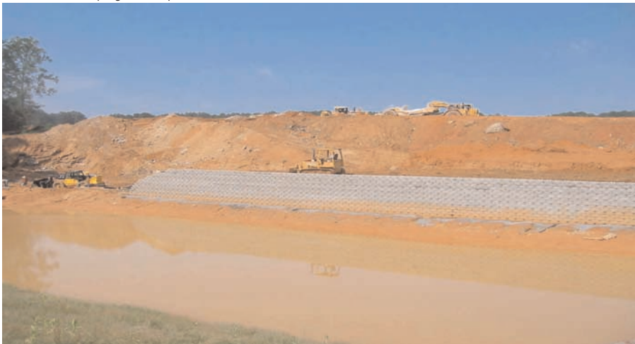
A one foot blanket drain, stone, and perforated pipe was placed behind the wall to allow sufficient drainage.
