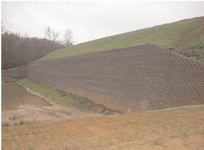
The completed wall was 30 feet tall and 300 feet long.
