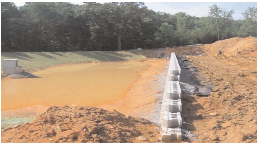
The base of this segmental retaining wall was reinforced with Miragrid® 10XT. Miragrid® 8XT, 5XT, and 3XT were used as the wall progressed upward.
