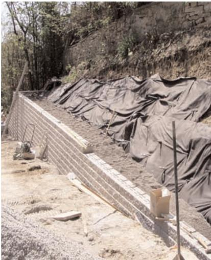
Wall under construction, showing earth anchors.
