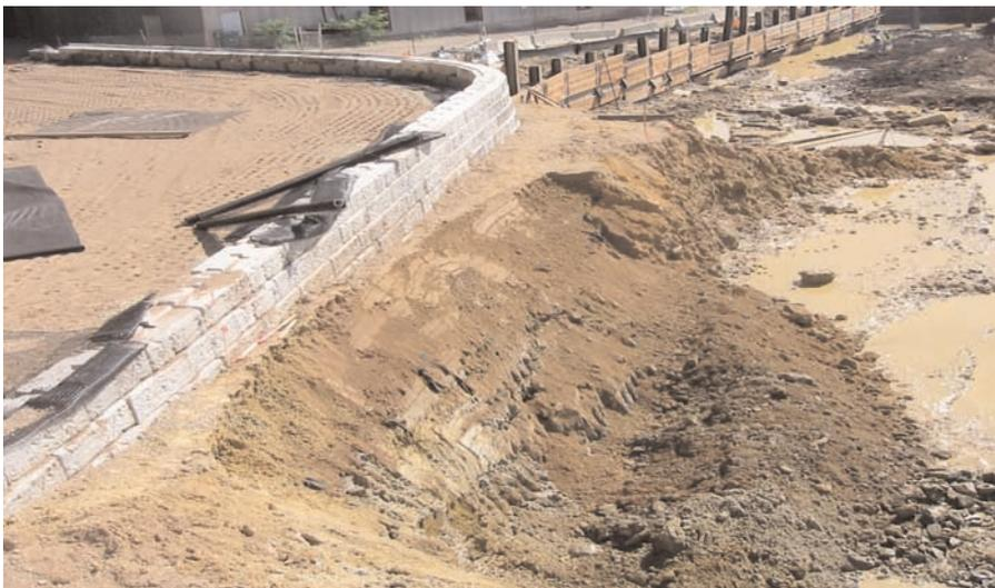
The design by CSG required that H-Piles be driven @ 6' O.C. into competent bedrock and capped with an H-Pile beam to support the retaining wall facing units in this area. Crushed stone was filled on top of the H-Pile beam up to the wall base elevation. The walls are currently under construction, and a September completion date is anticipated.
