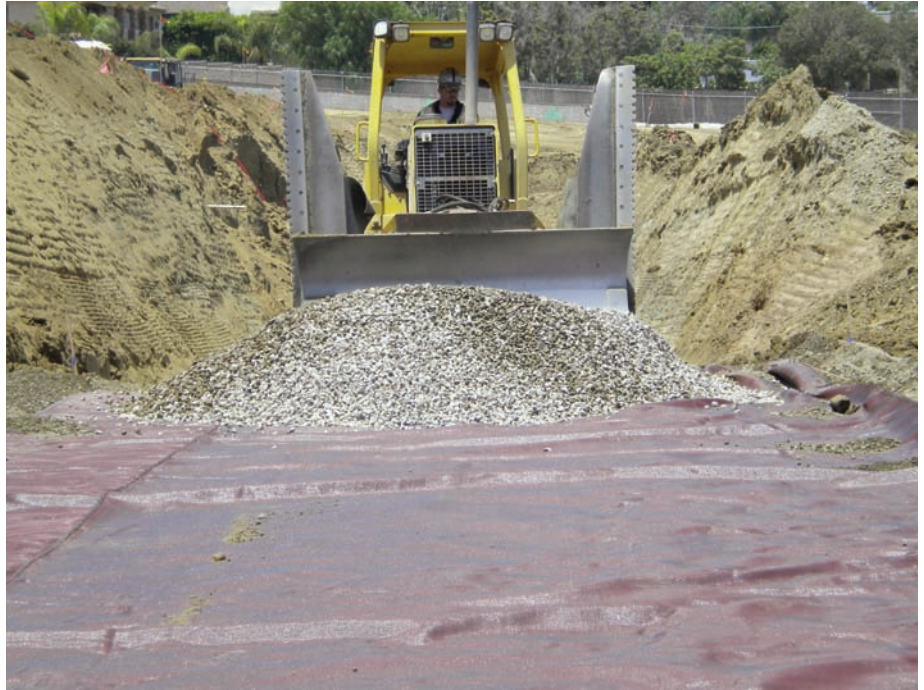
Base material being end dumped and spread on Mirafi® RS580i.
