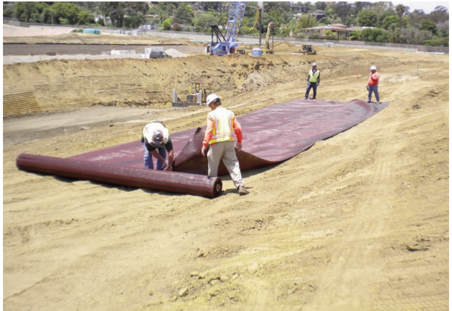
Preparation of Mirafi® RS580i material for placement.
