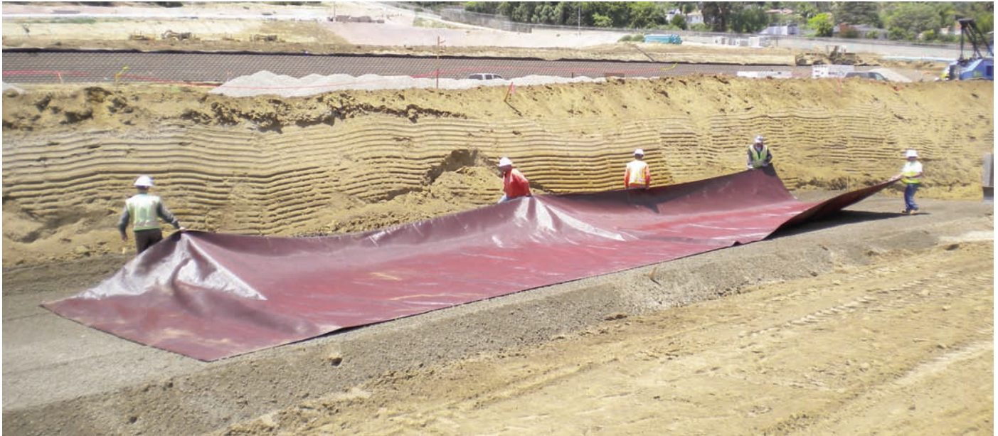
Installation of Mirafi® RS580i on soft soil area.
