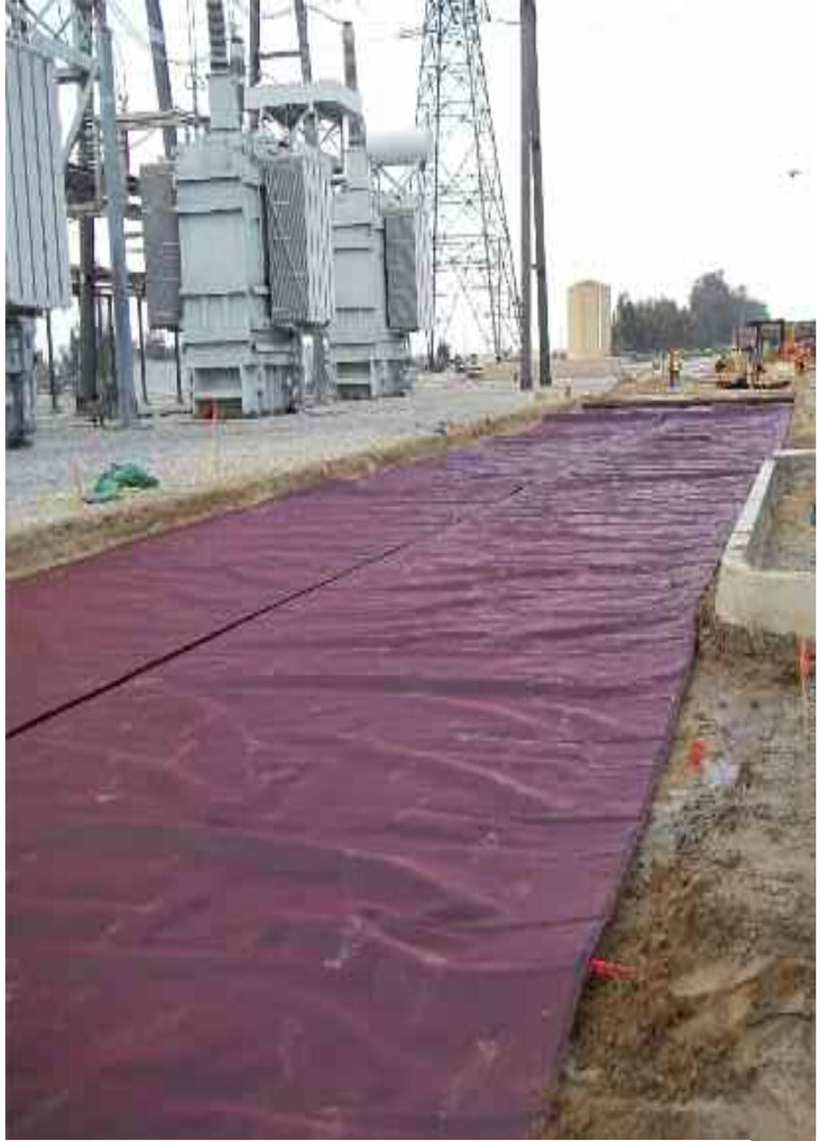
Mirafi® RS580i is rolled out across the poor subgrade before the base aggregate is added.
