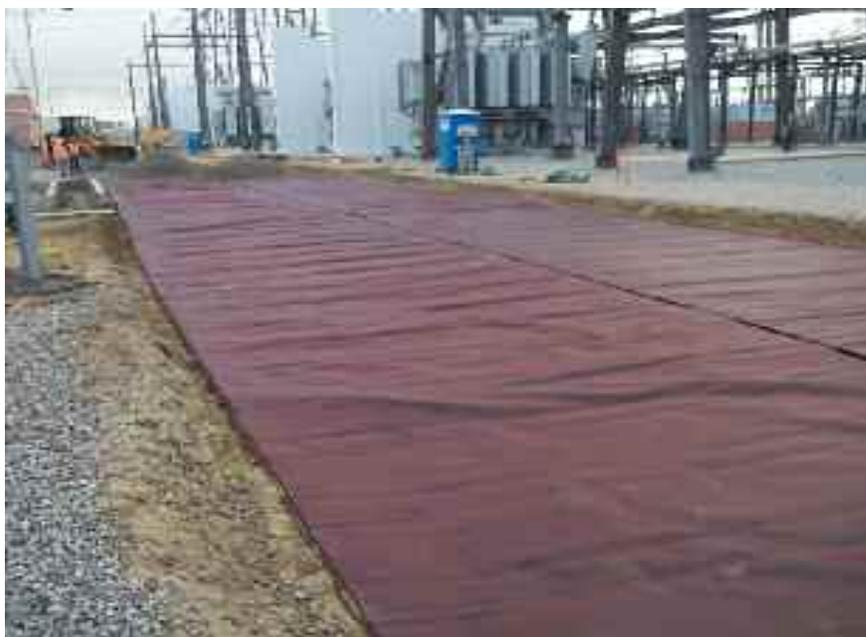
Dozers begin to place the aggregate material on top of Mirafi® RS580i.
