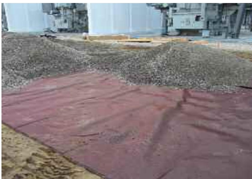
Aggregate is placed on Mirafi® RS580i and is ready to be spread evenly in preparation for compaction.
