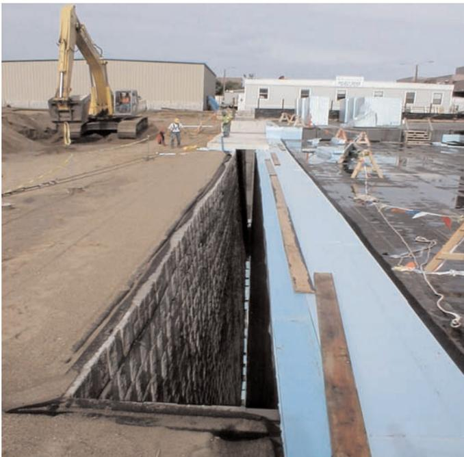
The mechanical connection of the Miragrid® - Anchor Landmark system enabled near a vertical stress relief wall.
