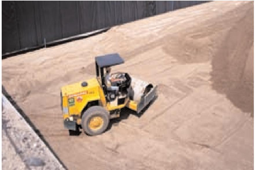
Miragrid® and granular fill were placed and compacted.
