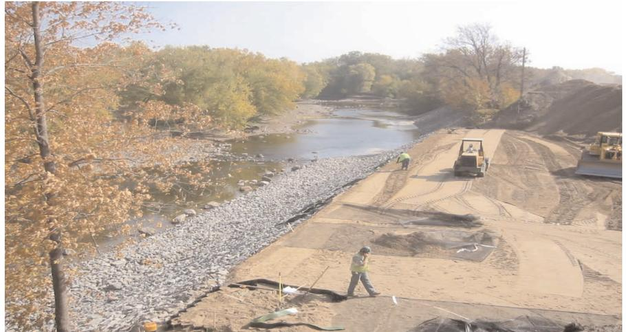
Deployment of Miragrid® geogrids as the embankment is half completed.
