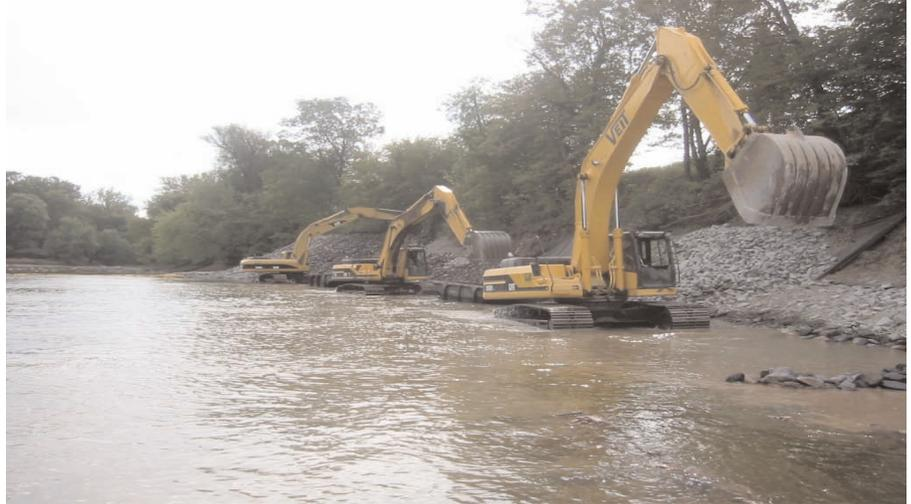
Placement of riprap on a granular filter over Mirafi® 180N during low river waters.
