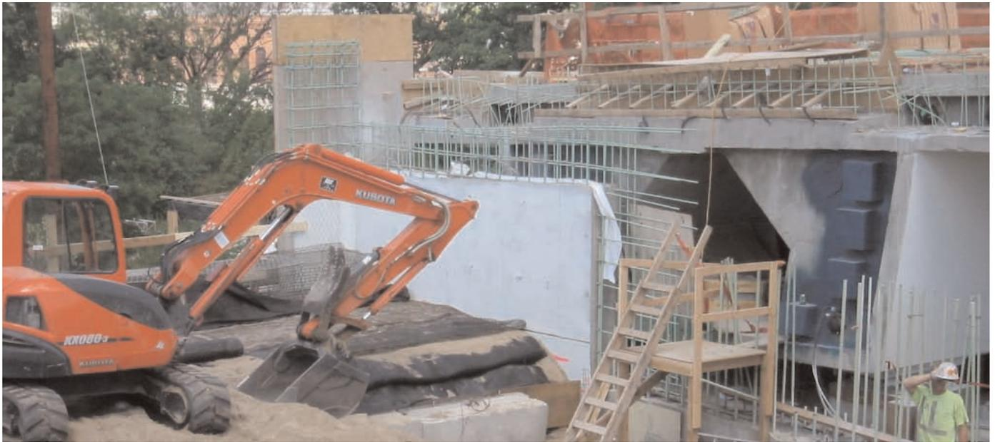
Temporary fabric wrapped wall at bridge abutment will allow Gabion retaining wall and bridge to be built concurrently.
