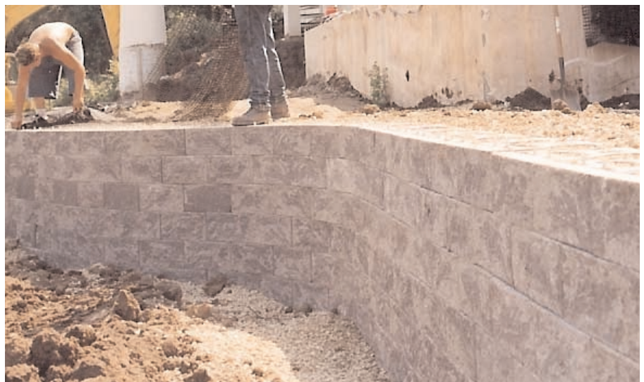
Installing geogrid for soil reinforcement.
