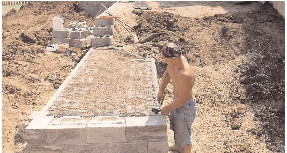
Connecting block and geogrid together.
