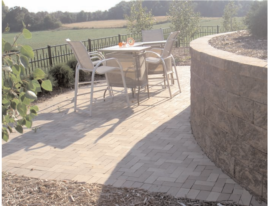
Above: Paver patio supported by reinforced block wall. Below: Amphitheater with fire pit completed.
