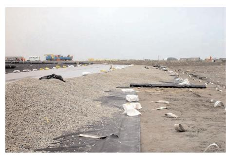
Rolls of Mirafi® BXG11 being deployed over areas of soft subgrade soil.
