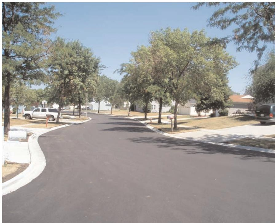
Thick paving fabrics such as Mirafi® MPV 700 are ideal for cold, harsh climates. The completion of Kensington Street with Mirafi® MPV 700 should delay reflective cracking.
