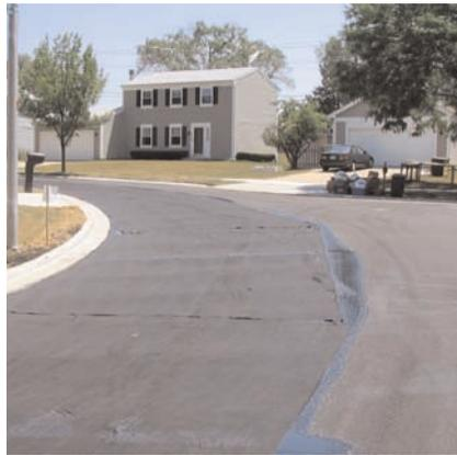
After the fabric is installed, pavement overlay was spread with 5cm (2in) of IDOT hot mix asphalt.
