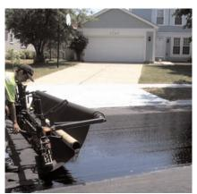
It is necessary to install the paving fabric in a timely manner when using a modified asphalt binder.
