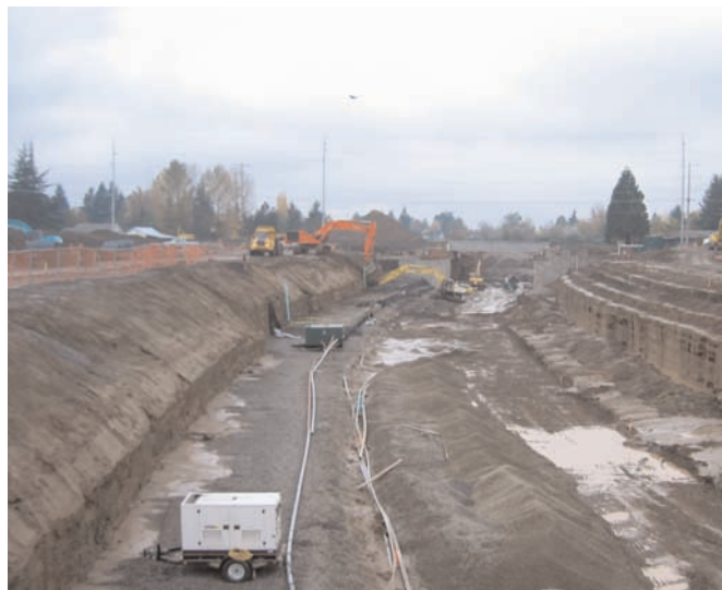
The beginning excavation of the lower roadway section.
