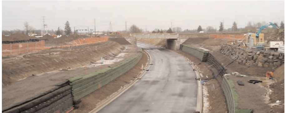
Above: The completed MSE walls without the other facing options. Below: The completed roadway with multiple MSE wall faces
