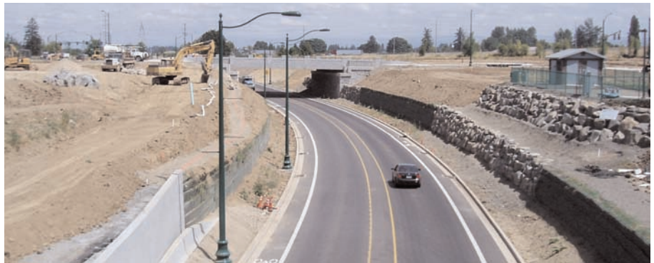
Above: The completed MSE walls without the other facing options. Below: The completed roadway with multiple MSE wall faces
