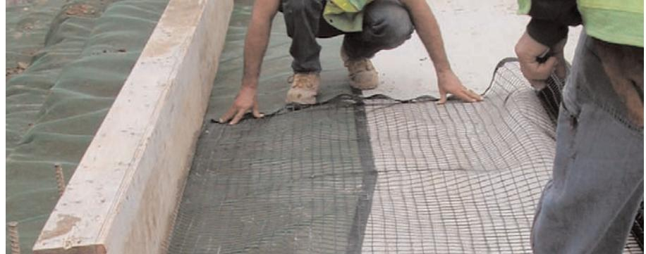
**Above:** Overlap required between primary reinforcement and face wrap.
