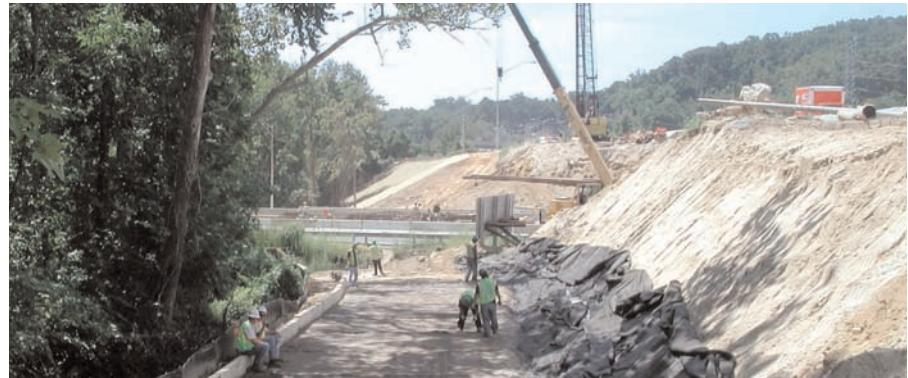
Preparing the drainage fabric behind the slope.
