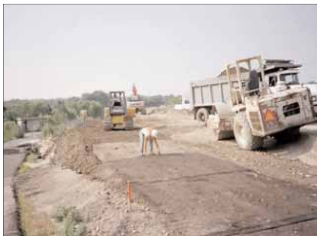
Miragrid® 8XT, used as the primary reinforcement, is installed in 0.9 m (3.0 ft) embedment lengths.
