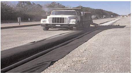
The trench was fitted with a 15.3cm (6in) HDPE pipe and backfilled with #57 stone.
