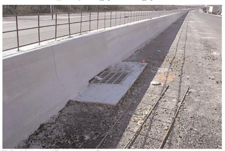
Median drains were used ffor stormwater runoff.
