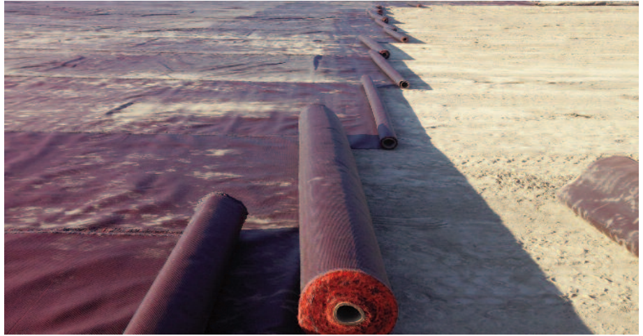
2 feet of overlap was need when placing the Mirafi® RS580i.
