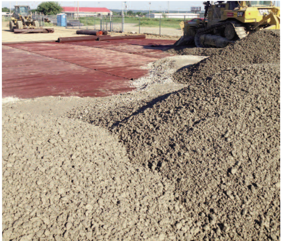
Bridging soft soils and building the platform.
