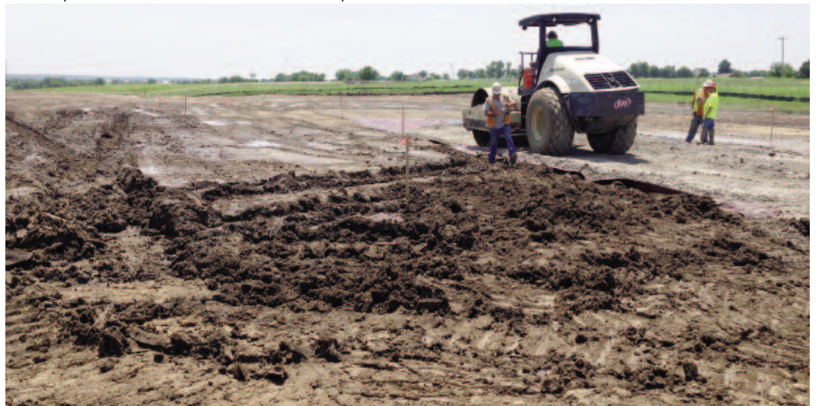
Working the subgrade before placement of Mirafi® RS580i geosynthetic.
