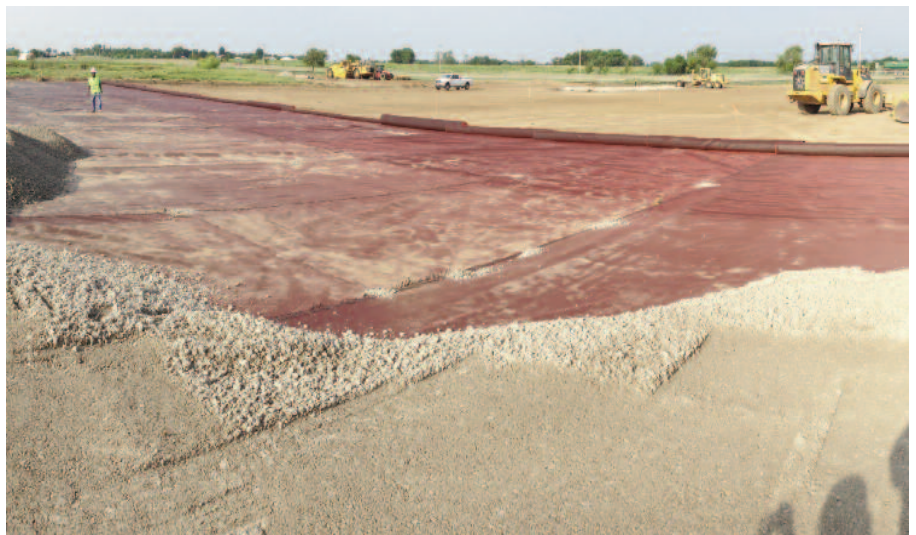
Blading out the aggregate on top of Mirafi® RS580i.
