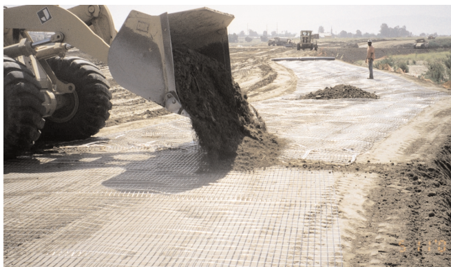
Enkagrid® PRO is placed in 3 foot intervals for a total slope of 20 feet. Enkagrid PRO was used to stabilize the slope under the water level.
