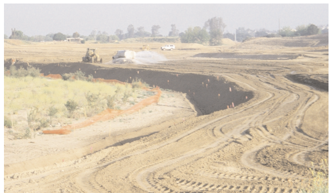
Enkagrid® PRO is placed in 3 foot intervals for a total slope of 20 feet. Enkagrid PRO was used to stabilize the slope under the water level.
