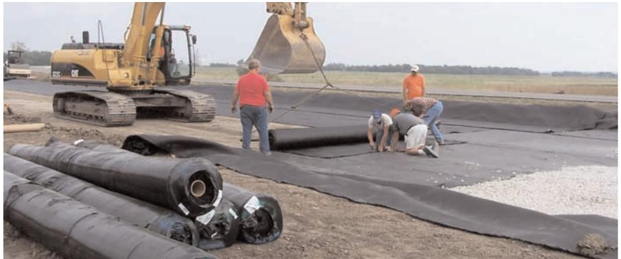
The Mirafi® HP570 is rolled out directly on the subgrade to stabilize the soft soils.
