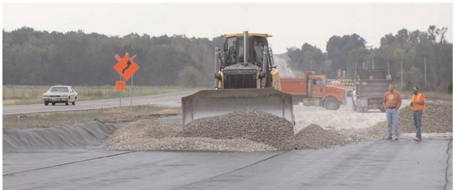
Base Rock is placed directly on the Mirafi® HP570.
