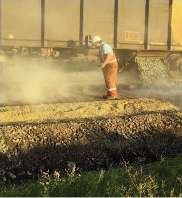
Placing new ballast.
