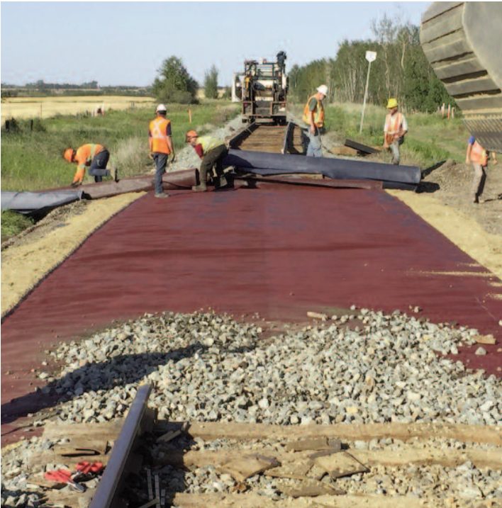
Mirafi® RS580i installed at the ballast/sub-ballast interface.
