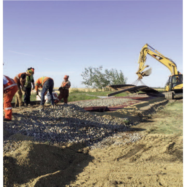
Reconnecting the track panel.
