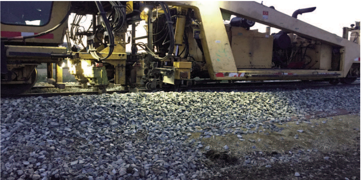
Lifting rail and compaction of ballast under rail ties.
