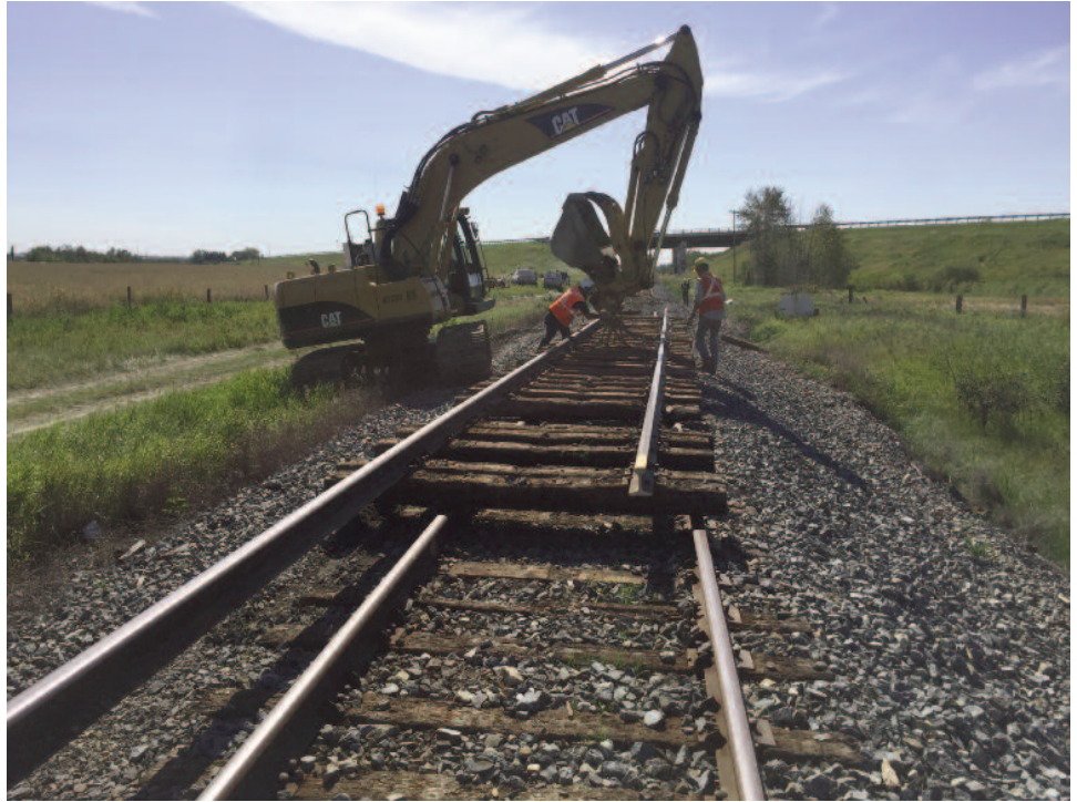
Track panel is removed.
