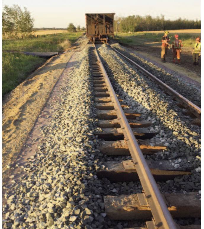
Placing new ballast.
