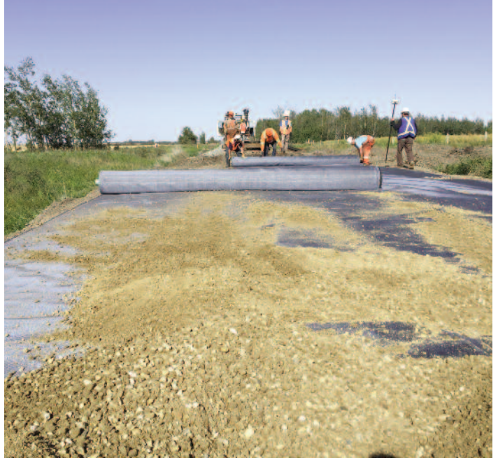
Mirafi® H2Ri installed at the subgrade/subballast interface.
