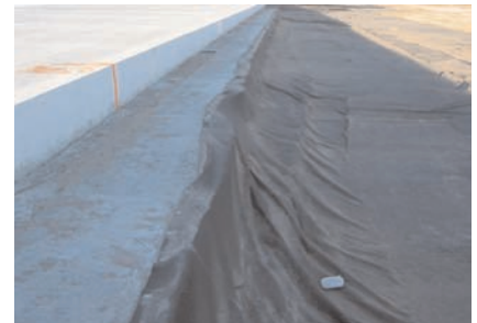
Mirafi® 170N was used for shoulder drainage.
