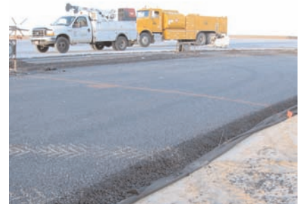
Mirafi® MPV 600 was used as a bond breaker.
