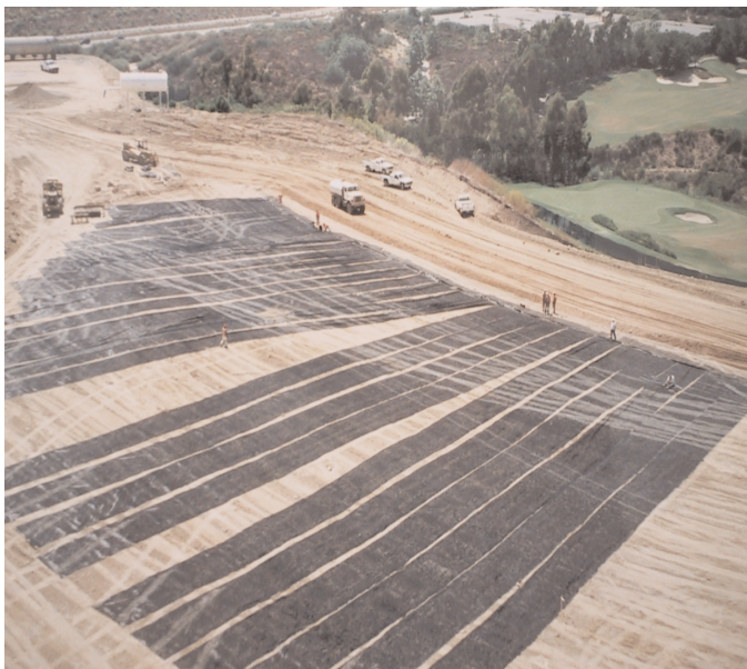
Over 400,000 yds 2 of Miragrid® geogrids were used to reinforce this development.
