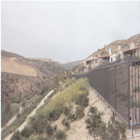
The slopes are now vegetated and look natural to the environment.
