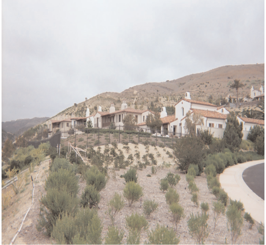
These premium lots were considered unbuildable. Miragrid® geogrids made it possible to develop this valuable property.
