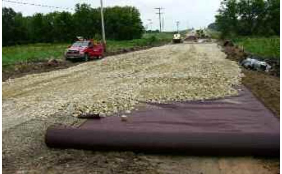
Installation of Mirafi® RS580i beneath 3" of rock.
