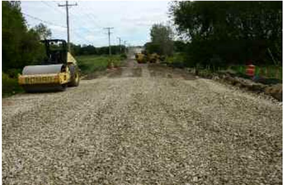
Construction continues upon completion of compaction. The revised cross section with Mirafi® RS580i passed proof roll.
