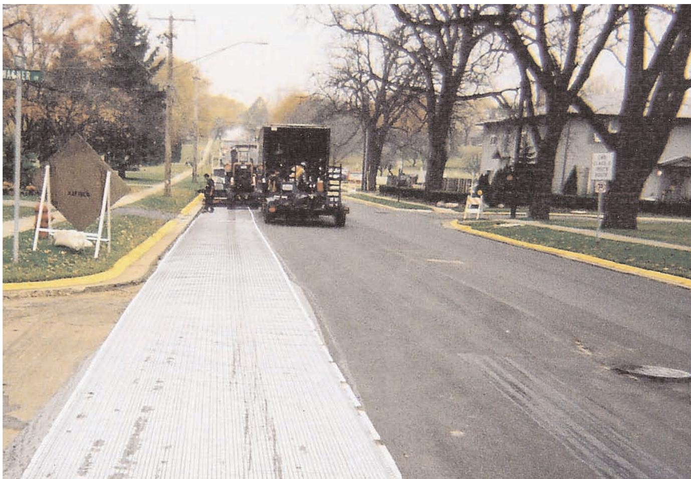
A light tack coat is spread to secure the Mirafi® FG to the binder course prior to pavement overlay.
