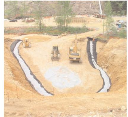
Base elevation with perimeter drain being installed.
