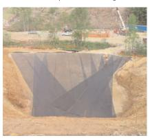
First layer of Miragrid® 24XT placed at base elevation.
