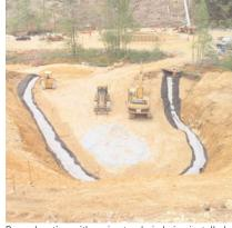
Base elevation with perimeter drain being installed.
