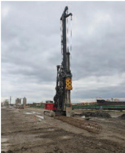
Driving piles on the reinforced platform.
