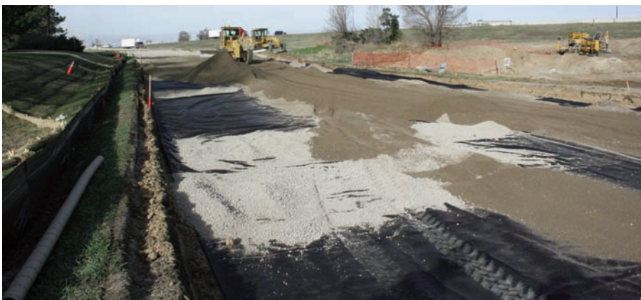
Placement of base material on Mirafi® RS580i.
