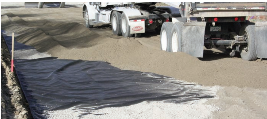
Base material being end-dumped on to Mirafi® RS580i.
