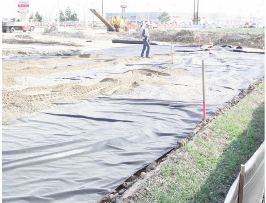
Placement of Mirafi® RS580i looking East .
