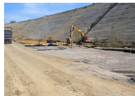
Construction of Miragrid® XT geogrid reinforced granular platform
