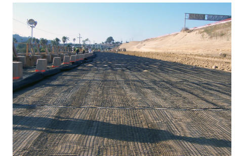
Placing Miragrid® XT geogrid reinforcement in the granular reinforced fill
