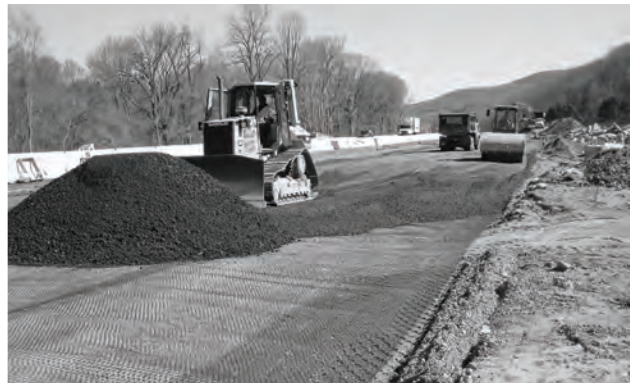
Image 9b: Spreading aggregate fill over Tensor Geogrid.
