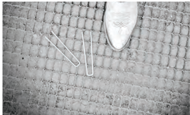
Image 7b: Staples for anchoring BX Geogrid (optional).
