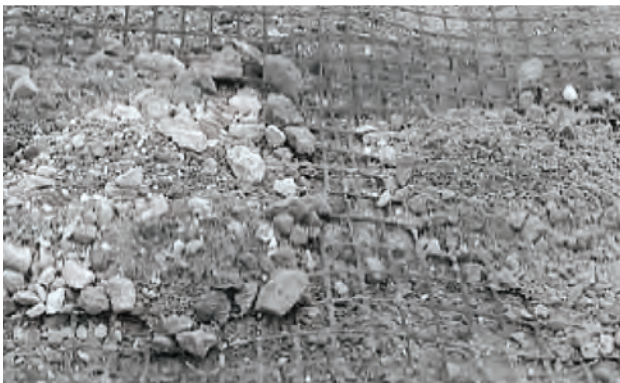
Image 7a: Anchoring geogrid with piles of aggregate.
