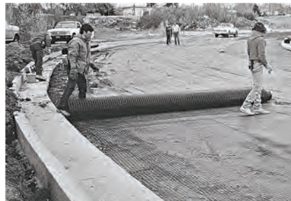
Image 5: Placing Geogrid to accommodate curves.
