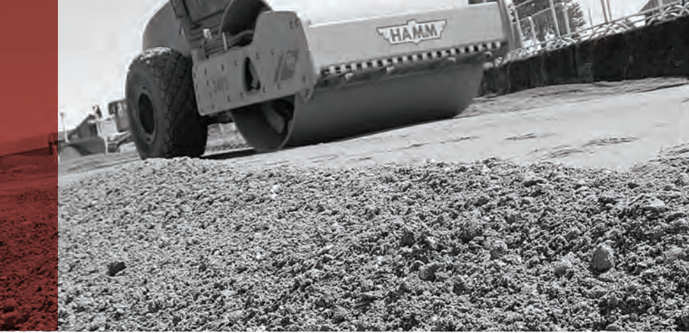
Image 11: Compacting the aggregate fill.
