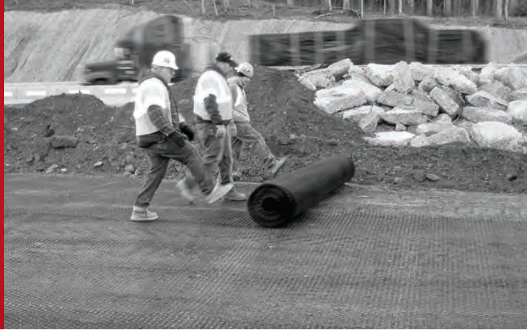
Image 3: Rolling out Tensor® Geogrid.
