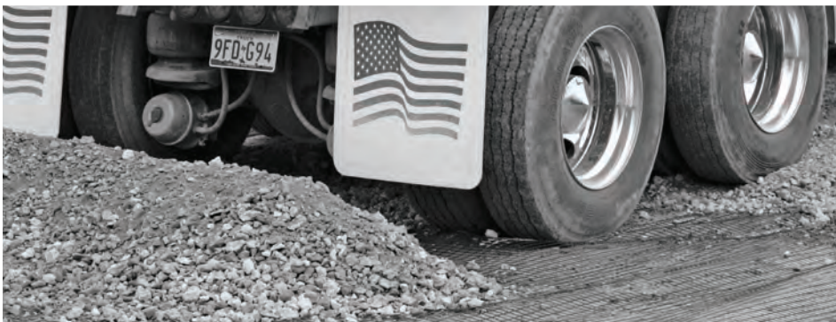
Image 12: Geogrid can be trafficked directly by rubber-tired equipment.
