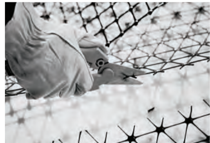
Image 6: Cutting Tensar® TriAx® Geogrid is easily achieved.
