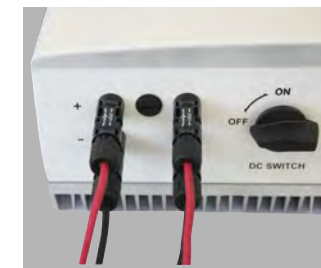
▲ Figure 4.12 Connect the DC Connectors to the Inverter
