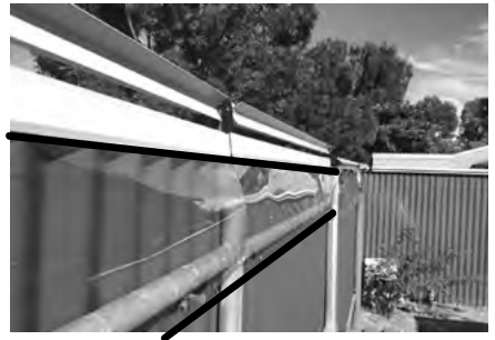
Clear polycarbonate sheeting installed just below Oscillot® eliminating the horizontal rail as a potential 'ladder'.
