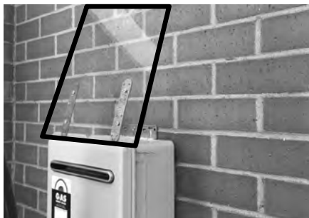
A rigid sheet of clear polycarbonate installed on an angle up to the wall preventing the cat from using the gas unit as a platform.
