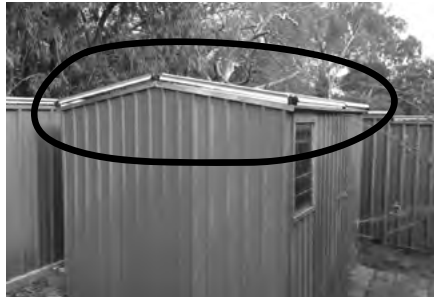
Oscillot® installed around shed roof perimeter to prevent cat from jumping on top of shed.
