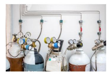
**Figure 5:** Typical high-pressure gas cylinders of nitrogen, helium, and oxygen (air zero) with gas pressure meters and regulators attached to piping lines that lead into a chemistry laboratory.
