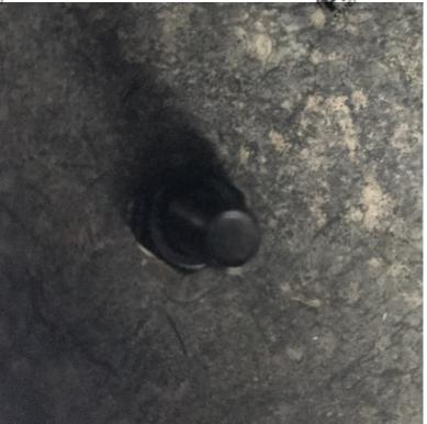
Reach under the mounting surface to screw the nut to your bolt.
