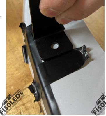
After lining this bracket up, take a sharpie or marker and marker the hole.
