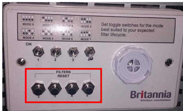
Filter Stage Reset Panel - FILTERS RESET
