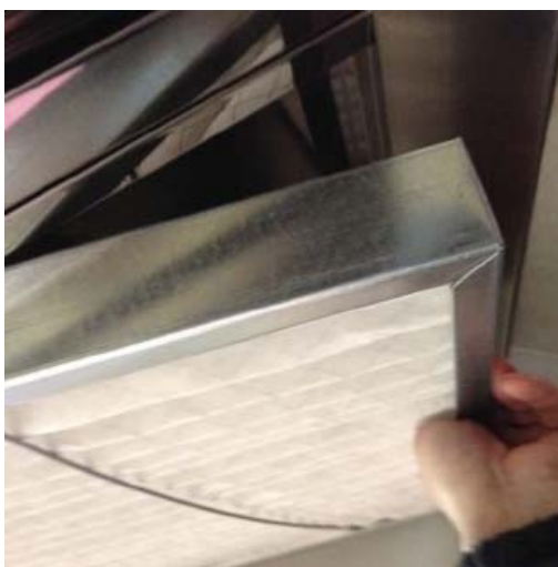
Removing the Stage 2 filter
