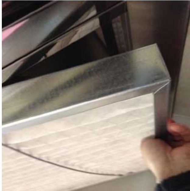
Removing the Stage 2 filter
