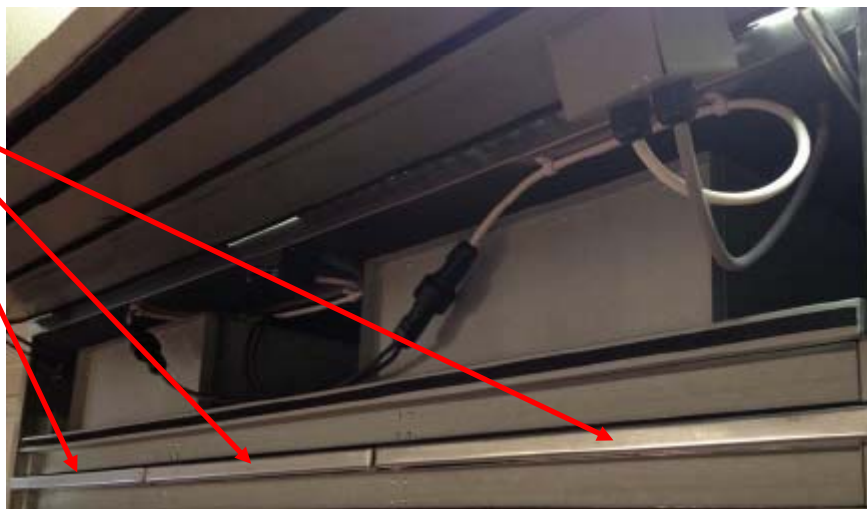
Stage 4 Replacing the Stage 4 Filters behind Access Panel
