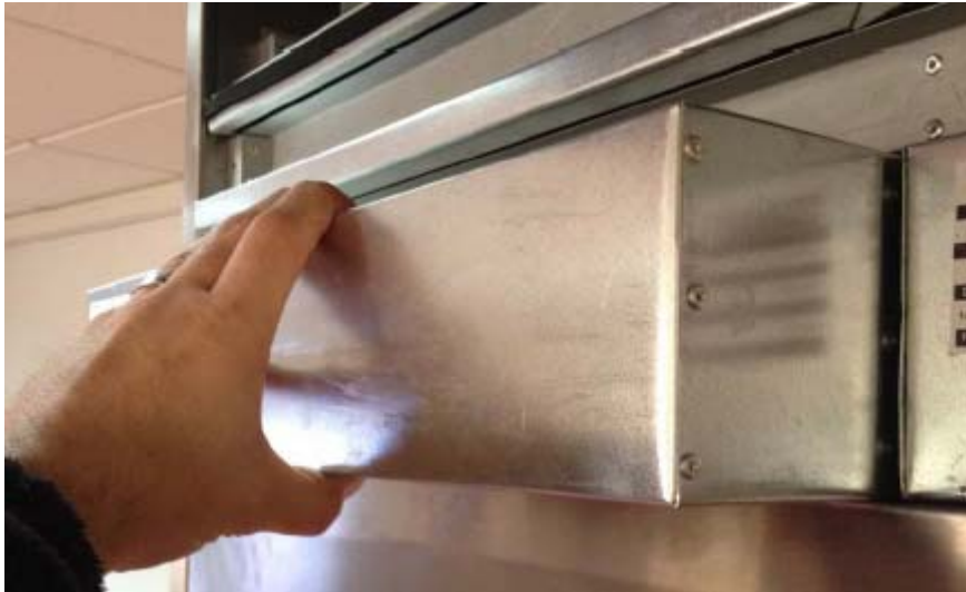
Sliding Back the Stage 3 Filter Panel
