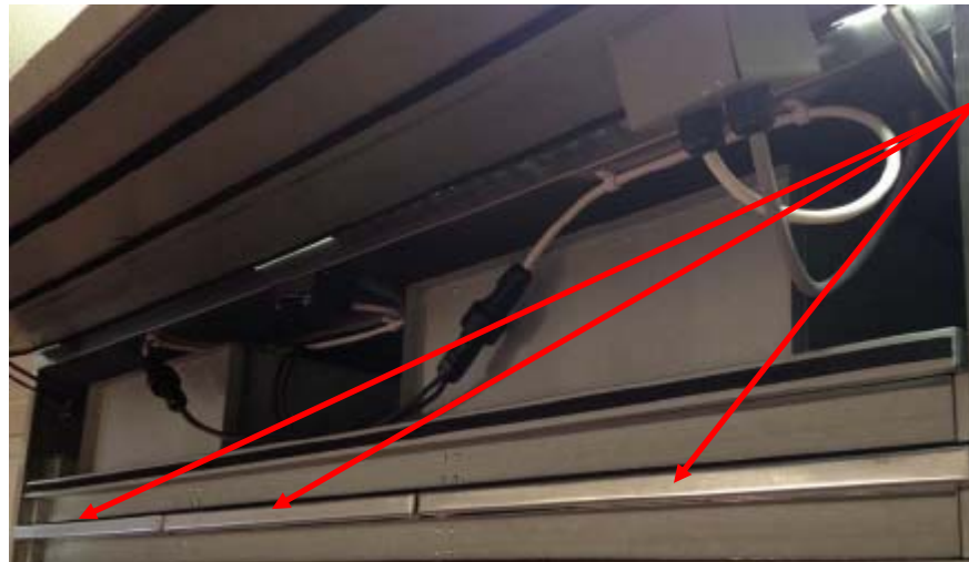
Stage 4 Carbon Filters Behind Access Panel
