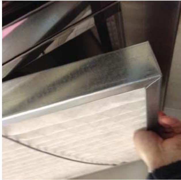
Replacing the Stage 2 Filter Panel
