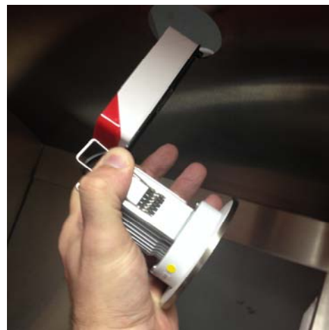
Removing the Fitting from the Canopy
