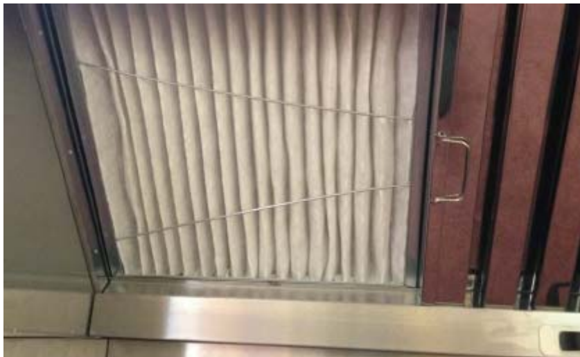
Stage 2 Filter Panel Replaced
