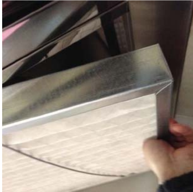
Removing the Stage 2 filter
