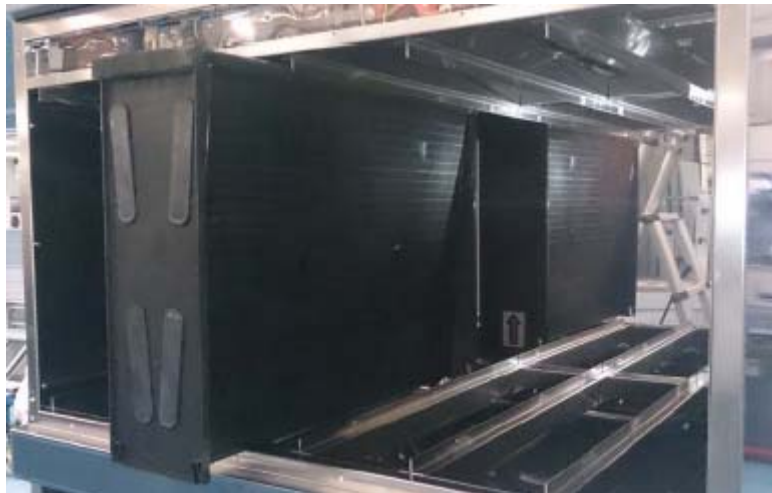
Removing Each of the Stage 5 Carbon Cells
