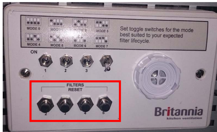
Filter Stage Reset Panel - FILTERS RESET
