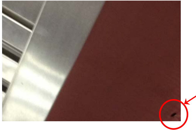
Grease Drainage Hole
