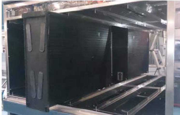
Replacing Each of the Stage 5 Carbon Cells
