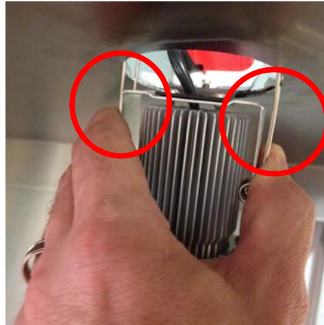
Squeezing the Spring Clips
