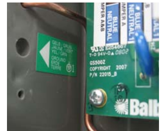
Ground in System Enclosure
