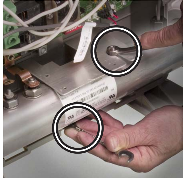
Remove both nuts that secure the element in place.
