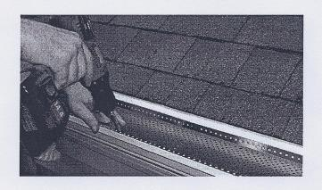
Shur Flo is designed to fit snugly under the drip edge against the back of the fascia. Shur Flo will perform well (most installations) without securing the panel to the fascia.
