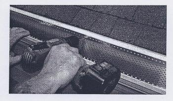
If the Shur Flo panel does not fit snugly, the panel may be secured by screwing a #10 x 1" screw through the back of the panel into the fascia. (#10 x 1" screws are included)
