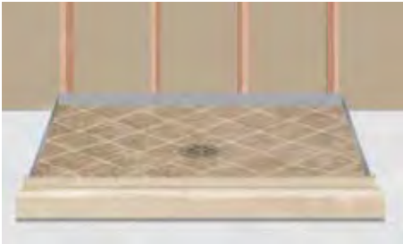
Install pan & drain
