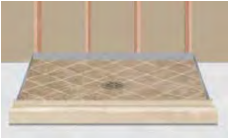
Install pan & drain
