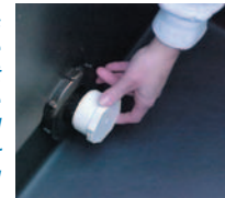
After both bulkheads are installed and the second hole is plugged, apply silicone to the PVC male adapter and turn into the bulkhead fitting. Be sure both pipe and fitting are free of dirt, then apply PVC primer to both followed by PVC glue. Insert pipe into fitting and allow to set for several minutes before burying.
