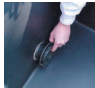
Install fitting with rubber gasket on the inside and the nut on the outside
