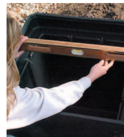
Be sure Aquafalls filter is level side to side and tipped forward ½" - 1".
