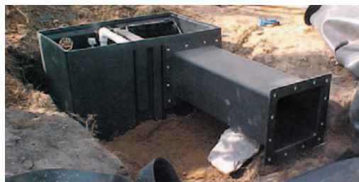
Be sure the opposite end of the extension tube is well supported with either compacted dirt or rocks.
