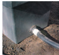
After both bulkheads are installed and the second hole is plugged, apply silicone to the PVC male adapter and turn into the bulkhead fitting. Be sure both pipe and fitting are free of dirt, then apply PVC primer to both followed by PVC glue. Insert pipe into fitting and allow to set for several minutes before burying.
